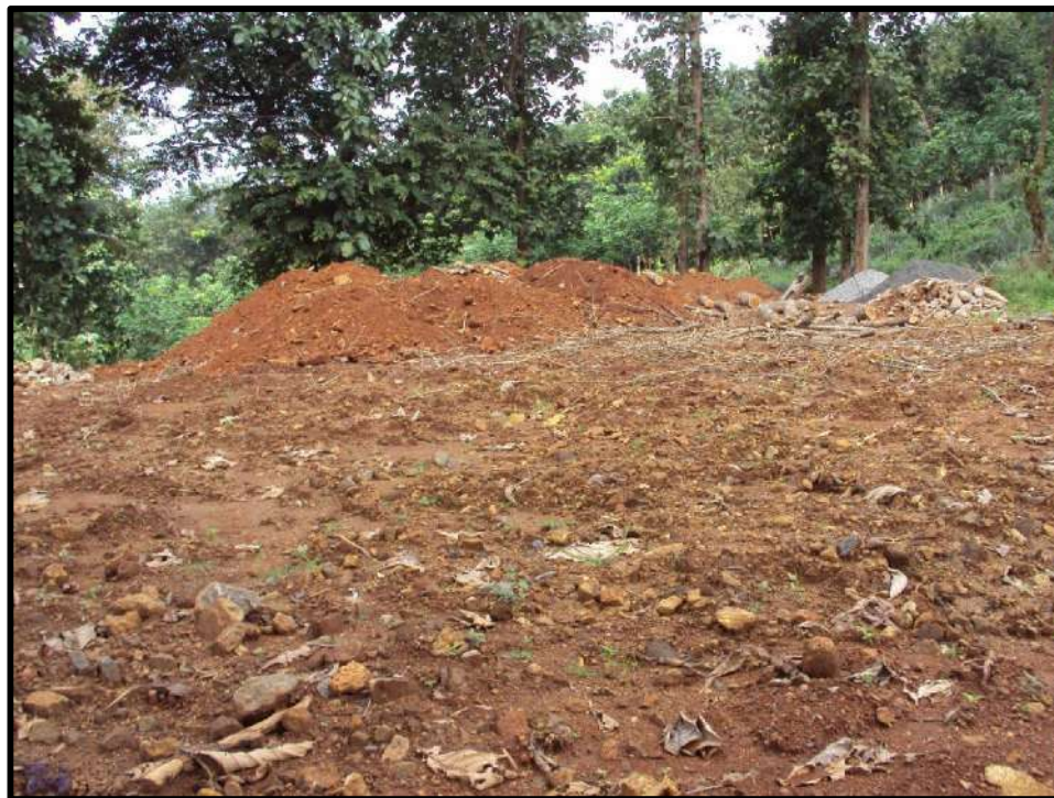
Photographs showing the top soil and OB storage area
