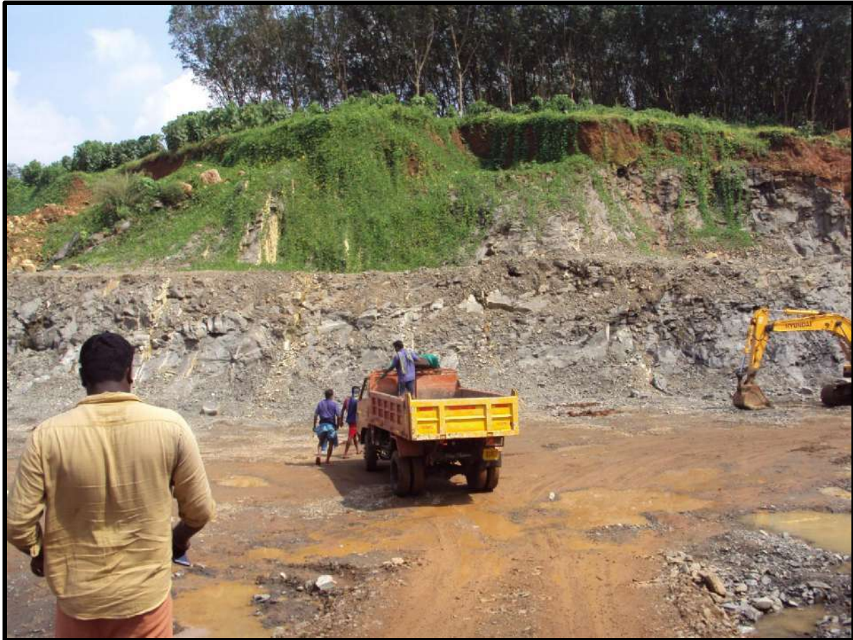
The photograph showing the starting of bench type mining
